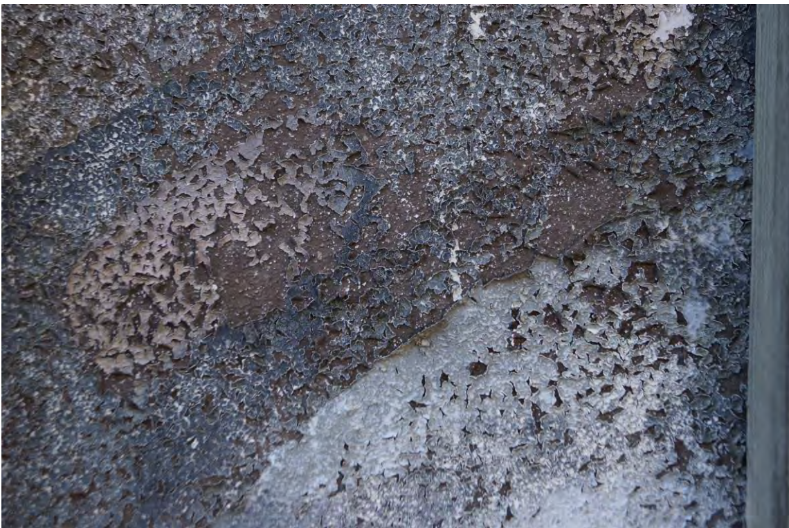
Images showing instances of extreme weathering to paint layers. Amongst them, fading, mildew and dirt build-up, extensive paint flaking and paint loss.
